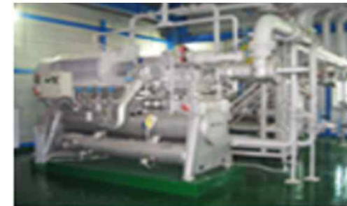
Tail Gas compressor
